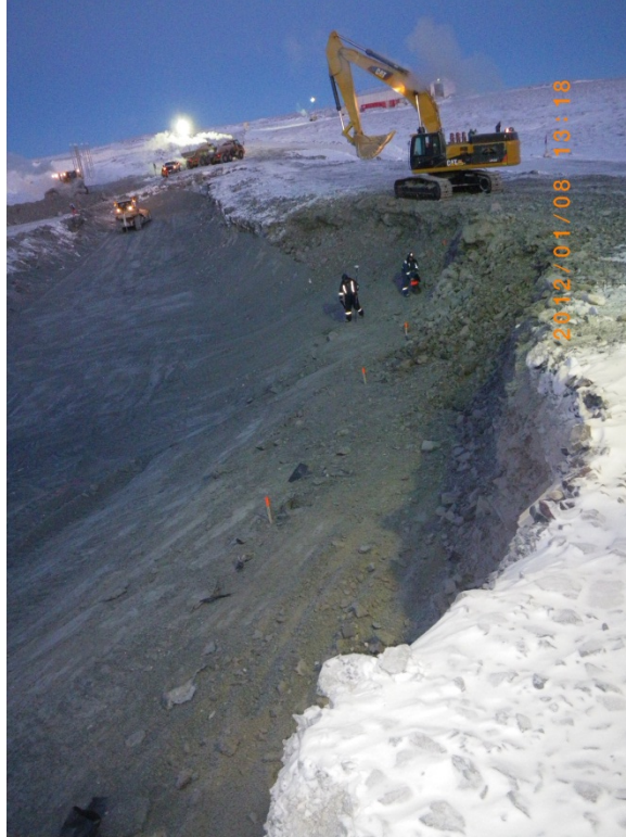
Photo 4: Exposed HDPE and GCL are shown in the foreground. At this point in time the extent of the damage is unknown.
