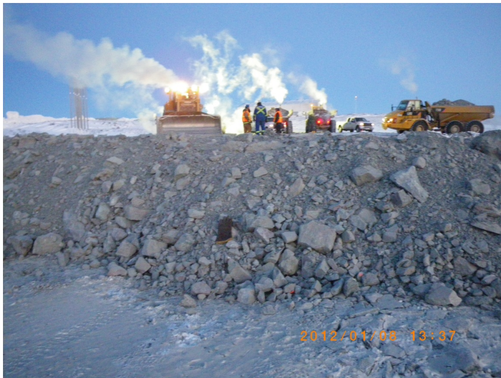
Photo 3: The blended material being placed in lifts within the downstream footprint of the dam.
