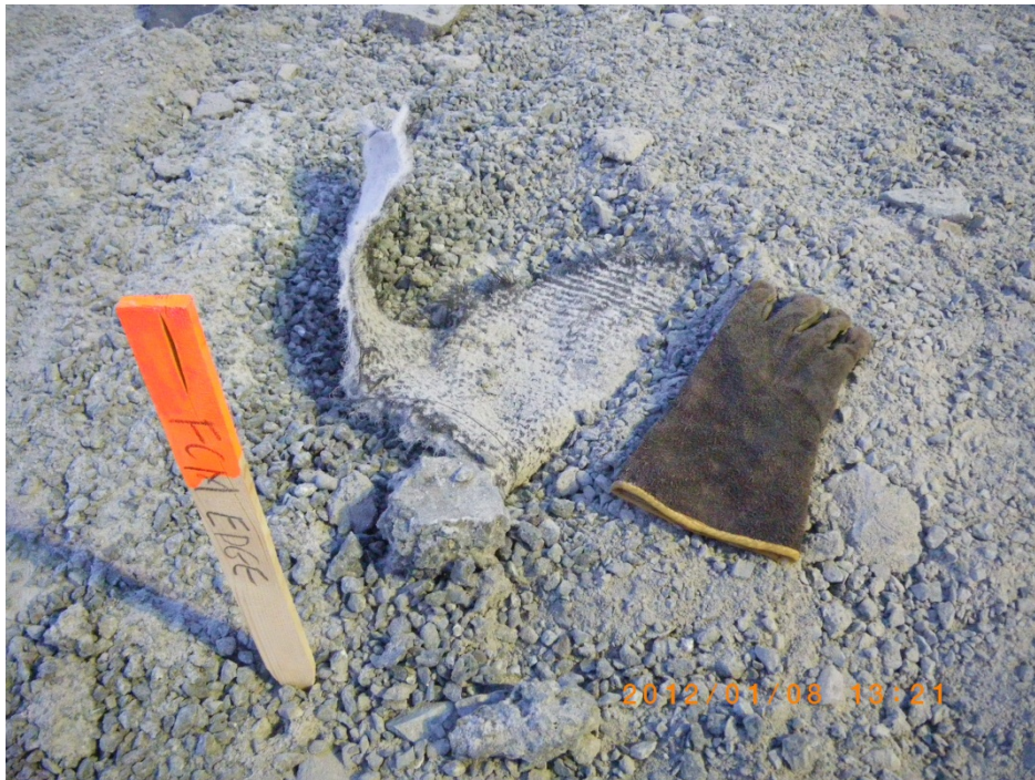
Photo 5: A closer inspection of the exposed GCL.
