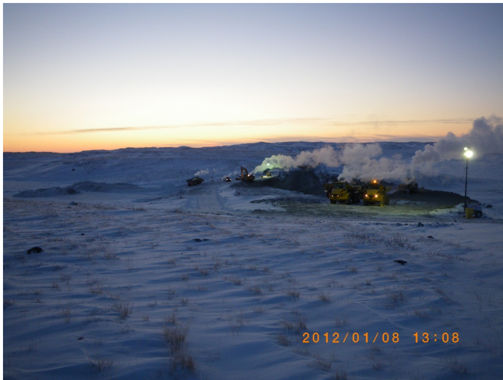
Photo 1: Removal of the 5/8" clear material and the ROQ from the upstream side of the keytrench. The mixed material is placed within the downstream footprint of the dam. The dirty snow pile, within Tail Lake, is visible on the left side of the photo.
